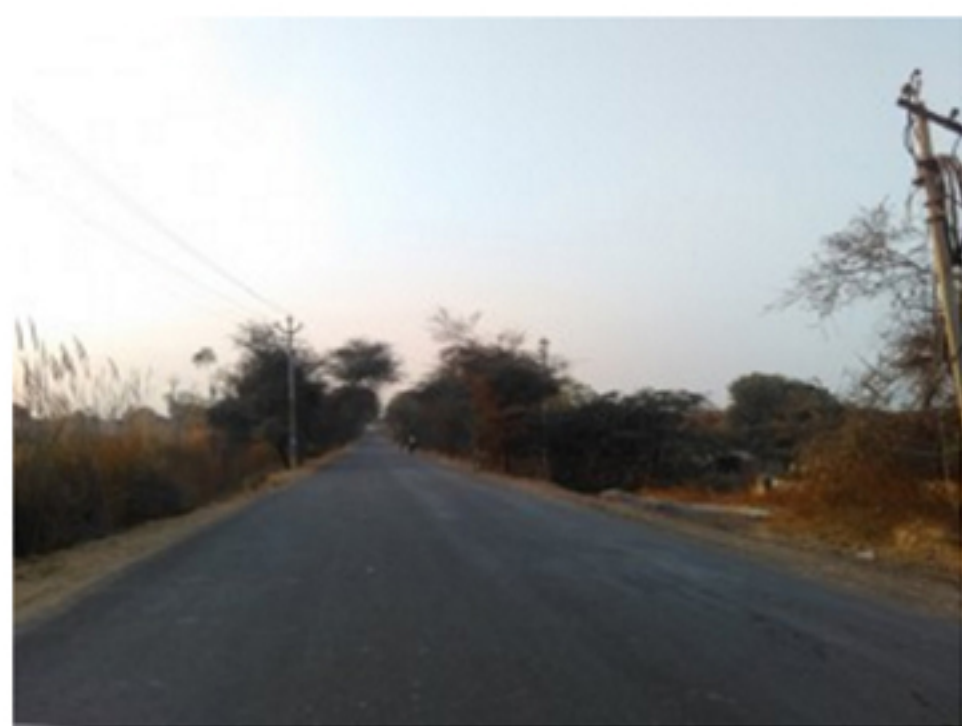
Current Road to Garhi Harsaru
